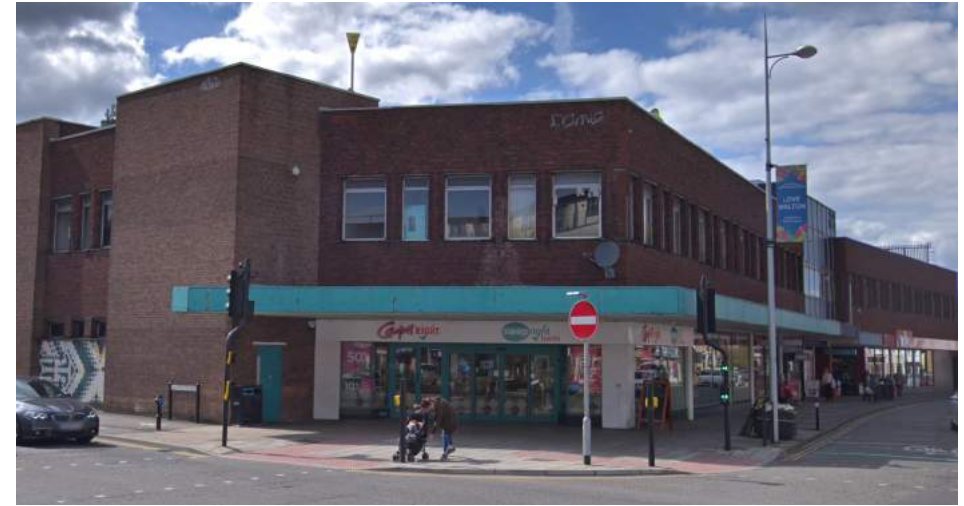
Street view of the existing building at the street corner showing the different brickwork panels and canopy
