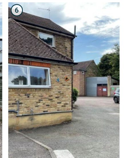
View of rear of Sundial House
