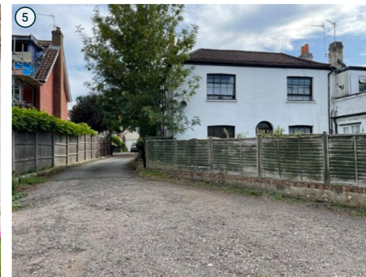
View of secondary access and Rivercroft House
