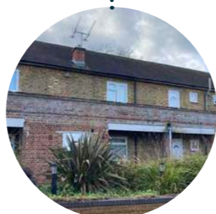
Horizontal parapets and white stone lintels
