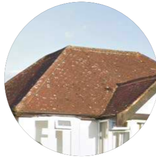
Hipped brown tiled roofs
