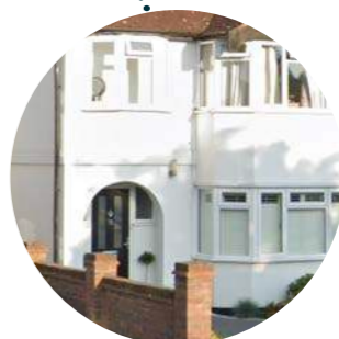
Covered entrances and rendered finishes
