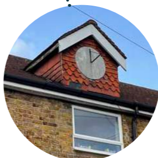
Circular roof features
