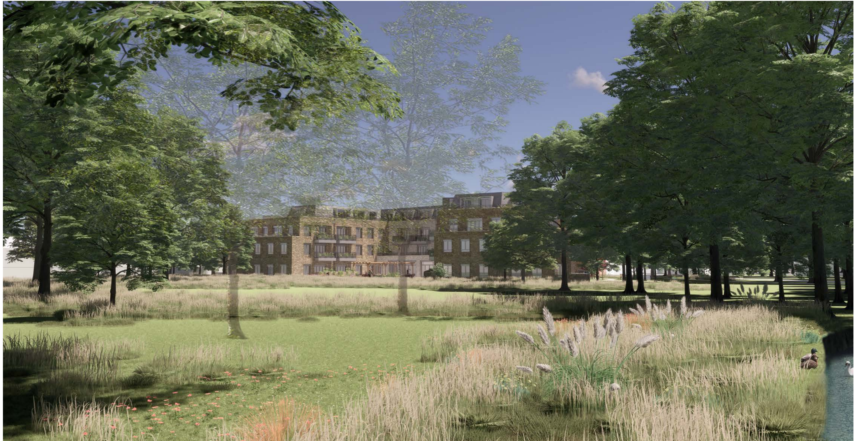
Building A view from private green belt land (some trees removed or faded to show building more clearly)
