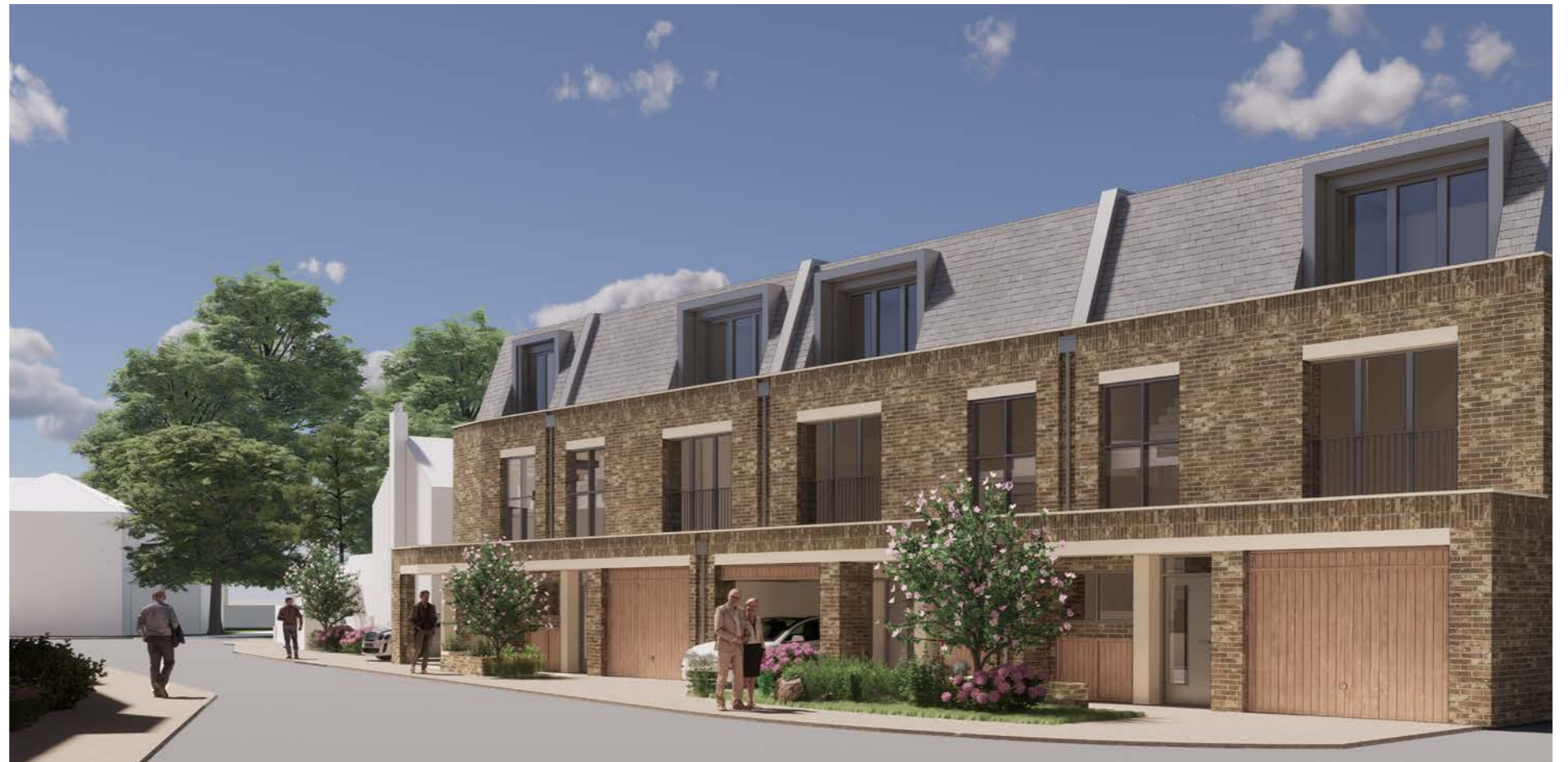
View towards building B - Mansard roof profile
