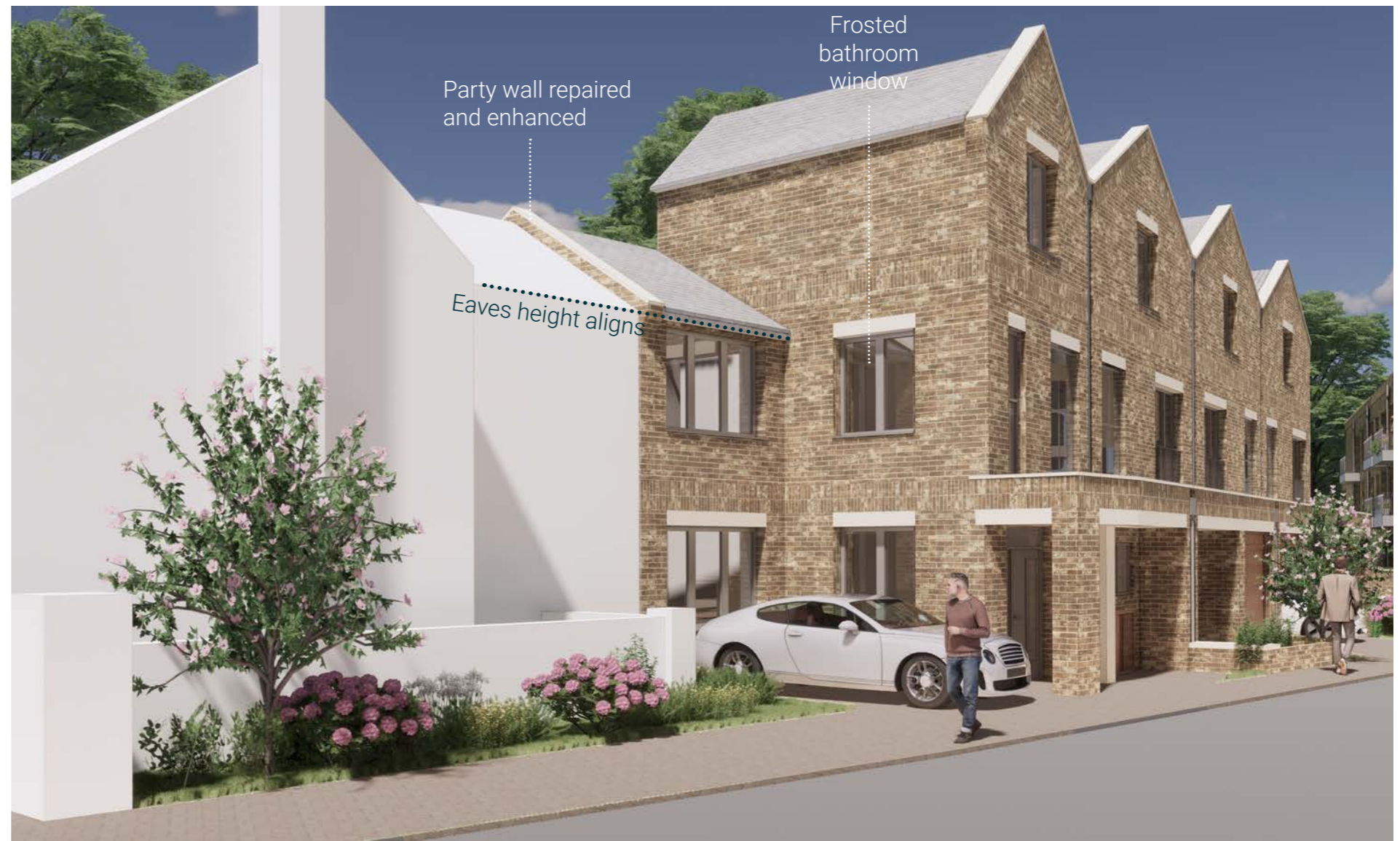
View towards building B and Ember Farm Cottage showing junction and alignment
