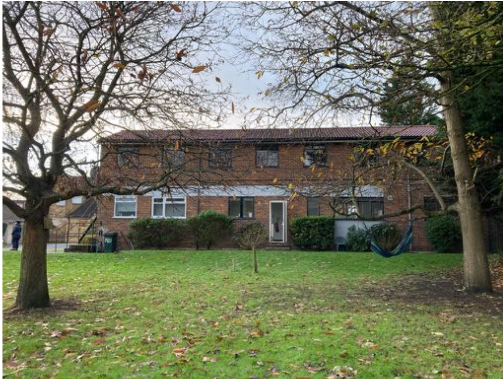
Photograph 11 Description: Rear (northern) elevation of The Molesey Venture accommodation Date: 08/12/2021 Location: View from northern Site boundary; looking to the south
