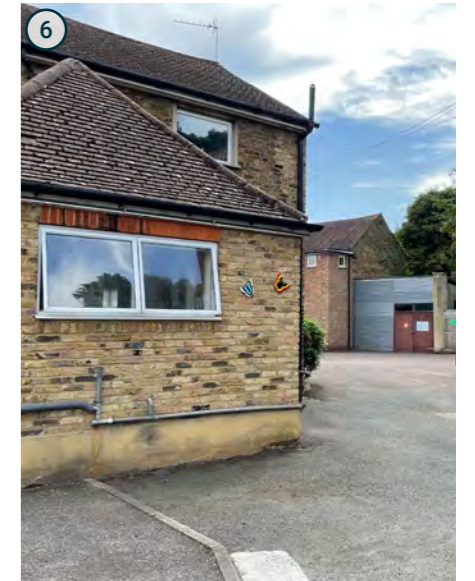
View of rear of Sundial House
