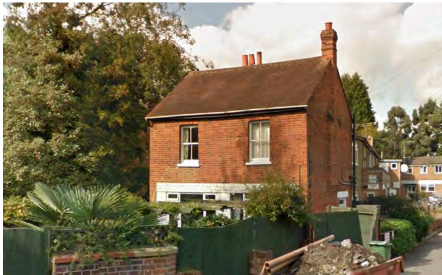
Ember Farm Cottage a two-storey cottage adjacent to the site
