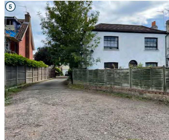
View of secondary access and Rivercroft House
