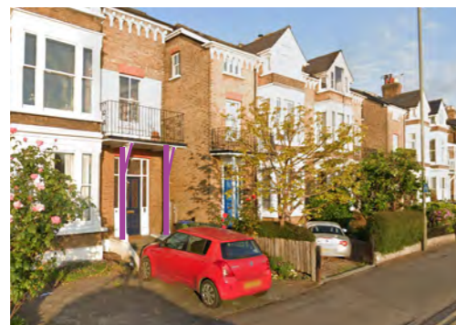
Local houses with projecting balconies and metal detailing
