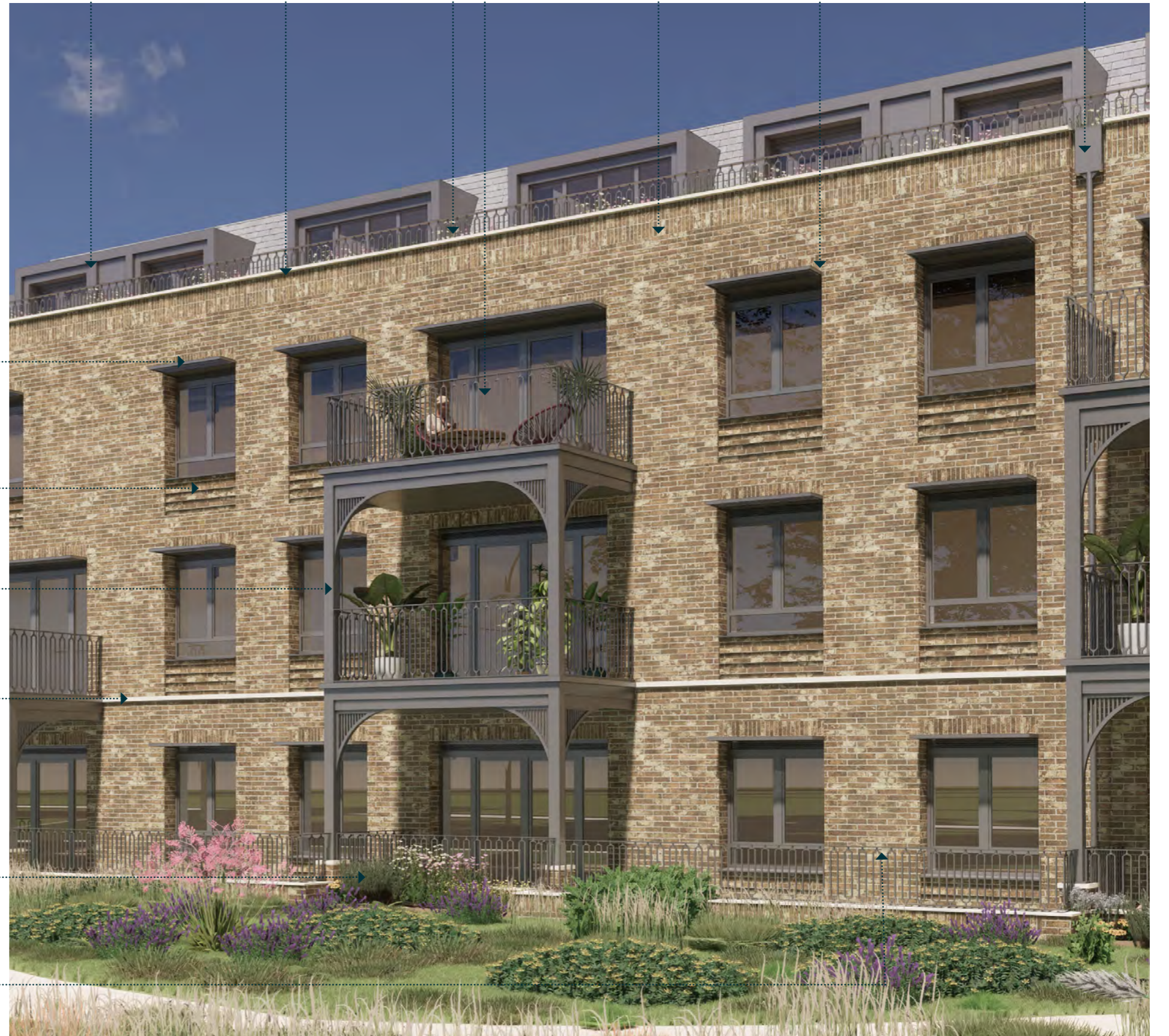
View from river towards Building A.
