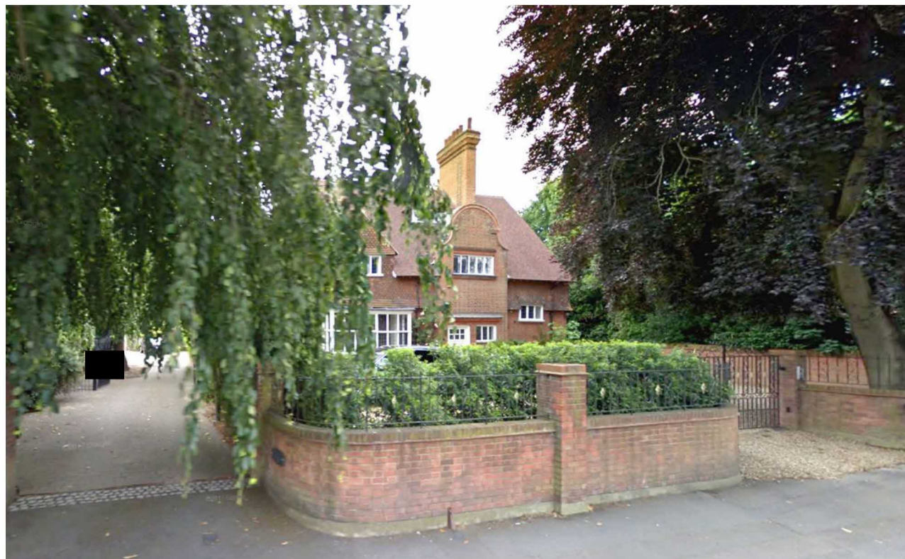
From Oatlands Drive looking east towards 1 Oatlands Drive
