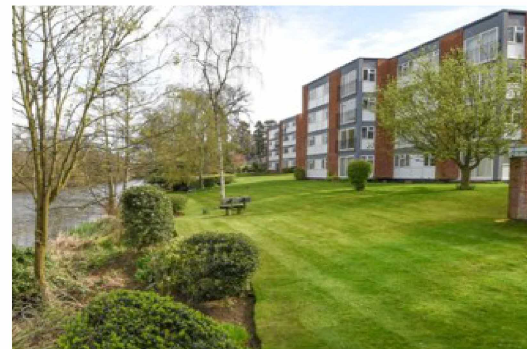
Berkeley Court - Rear elevation
