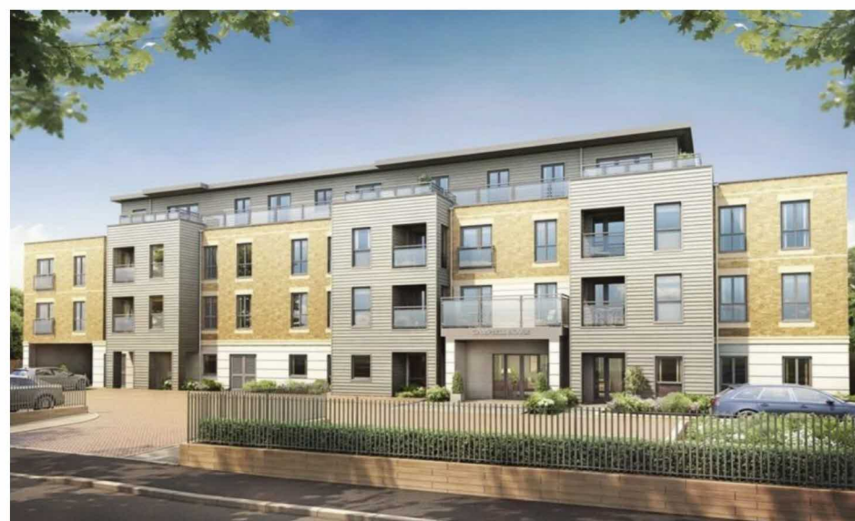
Campbell House, Queens Road, Weybridge
