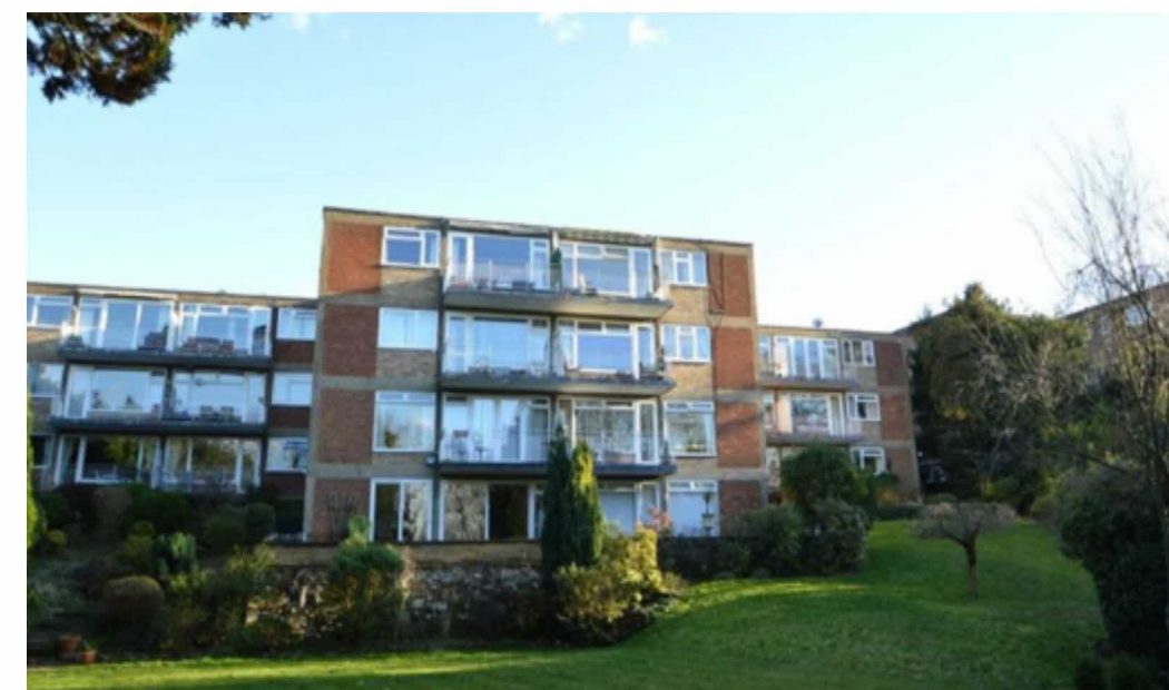
Chaseley Court, 42 Oatlands Drive - Rear elevation
