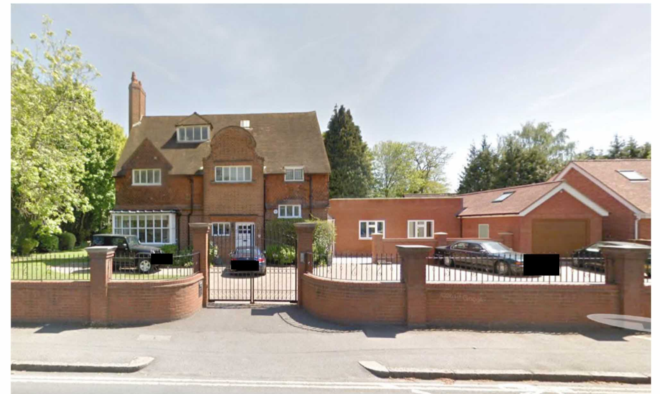
From Oatlands Drive looking east towards 3 Oatlands Drive
