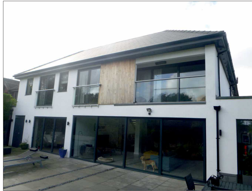
Photograph 6: Showing the rear of No.18.
