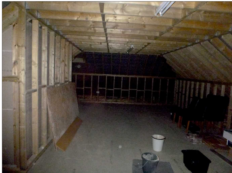
Photograph 7: Showing the roof space of No.18.
