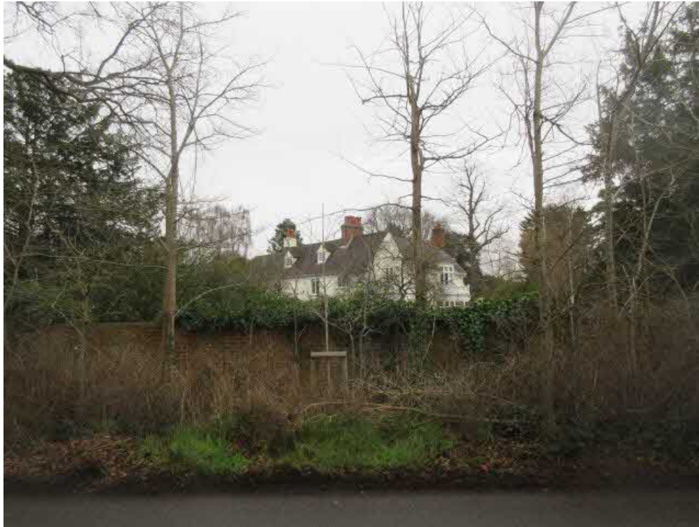
Plate 7: The Orchard, looking north east
