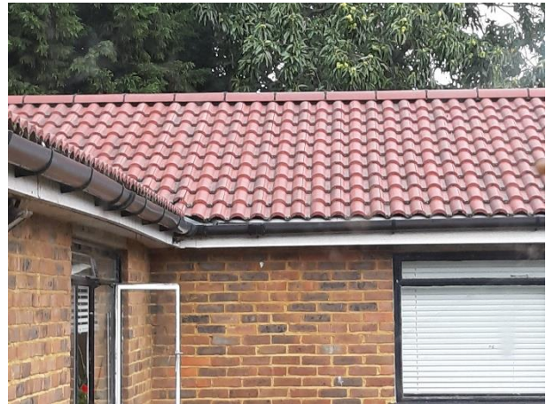
Plate 4.2: Clay Roof Tiles, B1
