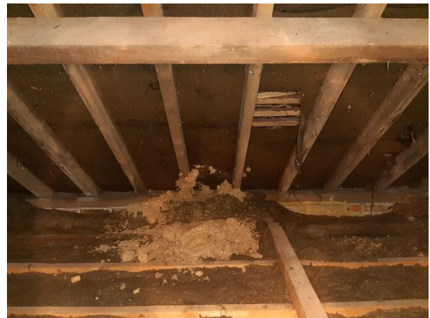
Plate 4.10: Torn Felt Sarking & Wasp Nest
