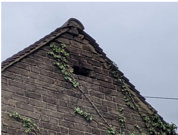
Plate 4.7: North-facing Gable End, B2
