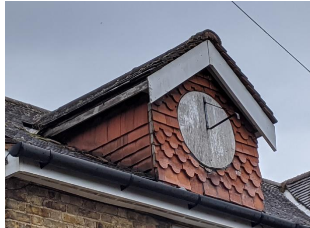
Plate 4.12: Hanging Tile Feature, B4
