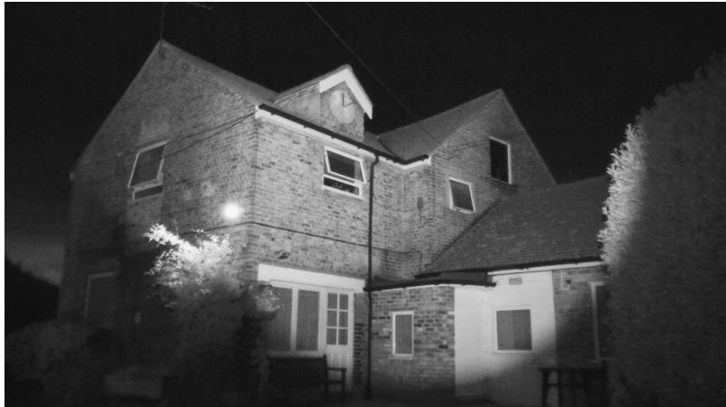
Plate 4.3.1 Screenshot of camera focused on Building 2 at 3:26am on the Dawn-Re-entry Survey 15/07/2022
