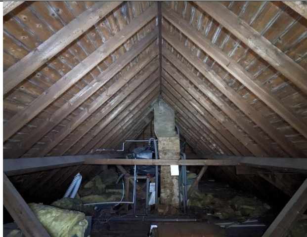
Photograph 5: Large loft void
