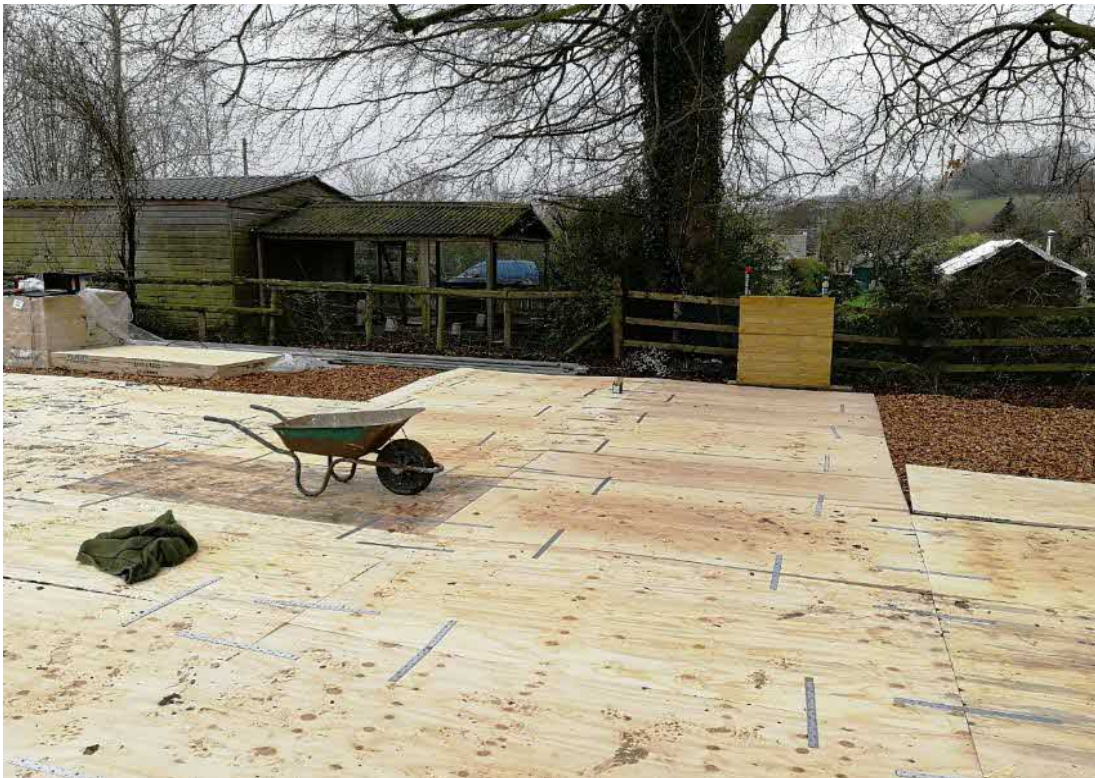
Figure 6 – Plywood sheeting used as ground protection.
