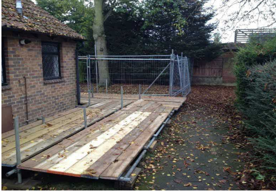
Figure 7 – Specification for scaffold ground protection.
