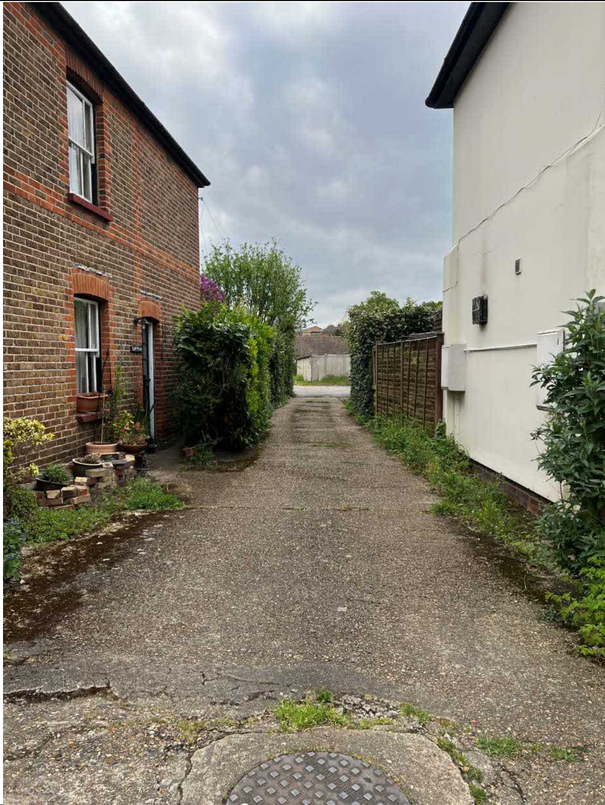
Photo 7: View of drainage location in access road
