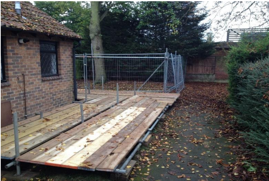
Figure 7 – Specification for scaffold ground protection.
