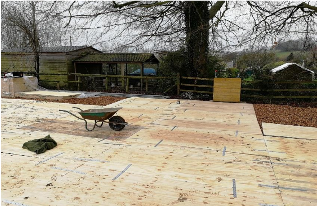
Figure 6 – Plywood sheeting used as ground protection.
