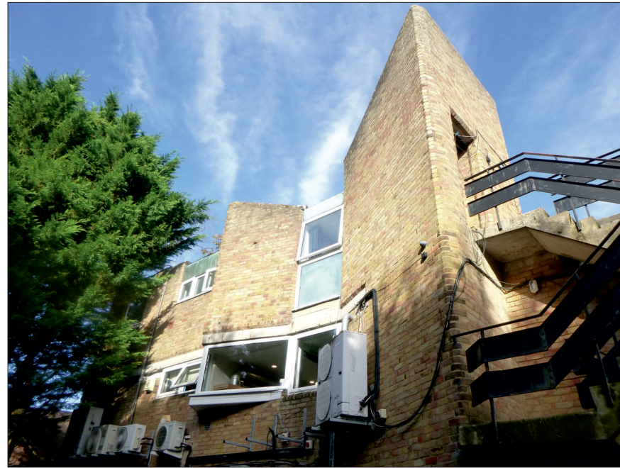
Photograph 2: Showing the rear of the buildings.
