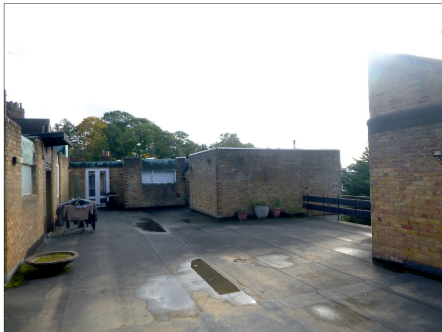
Photograph 3: Showing the flat, felted roof used by residents.
