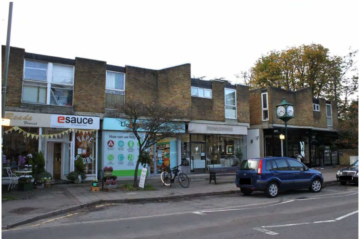
Figure 27 Plate 6 View to the Heath Buildings (west side) of the High Street (north end), looking north-west
