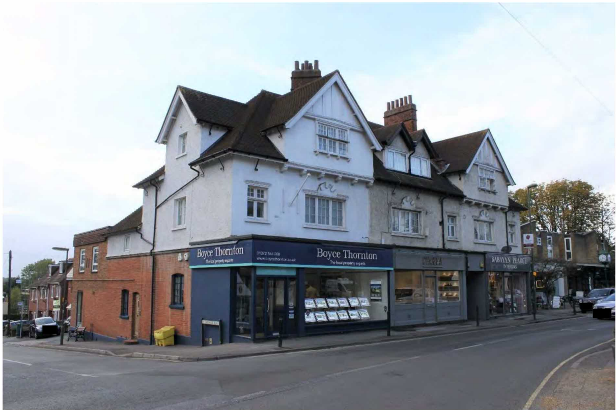
Figure 33: Plate 12 View to the buildings on the corner of Oakshade Road and the High Street and the south end of Heath Buildings, looking north-west
