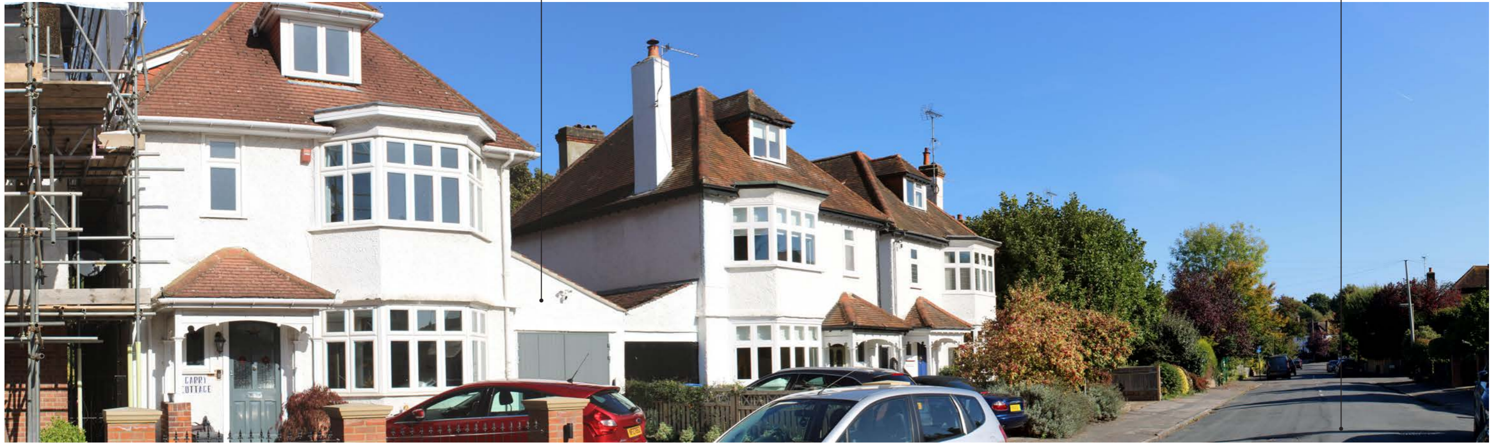
Photograph 15a View from Raleigh Drive looking north east (November 2022).
