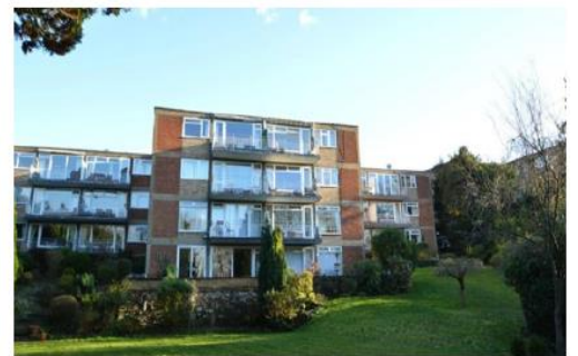
Chaseley Court, 42 Oatlands Drive - Rear elevation
