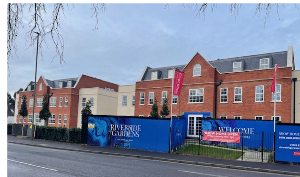
Riverside Gardens, 8-14 Oatlands Drive - Oatlands Drive elevation (under construction)
