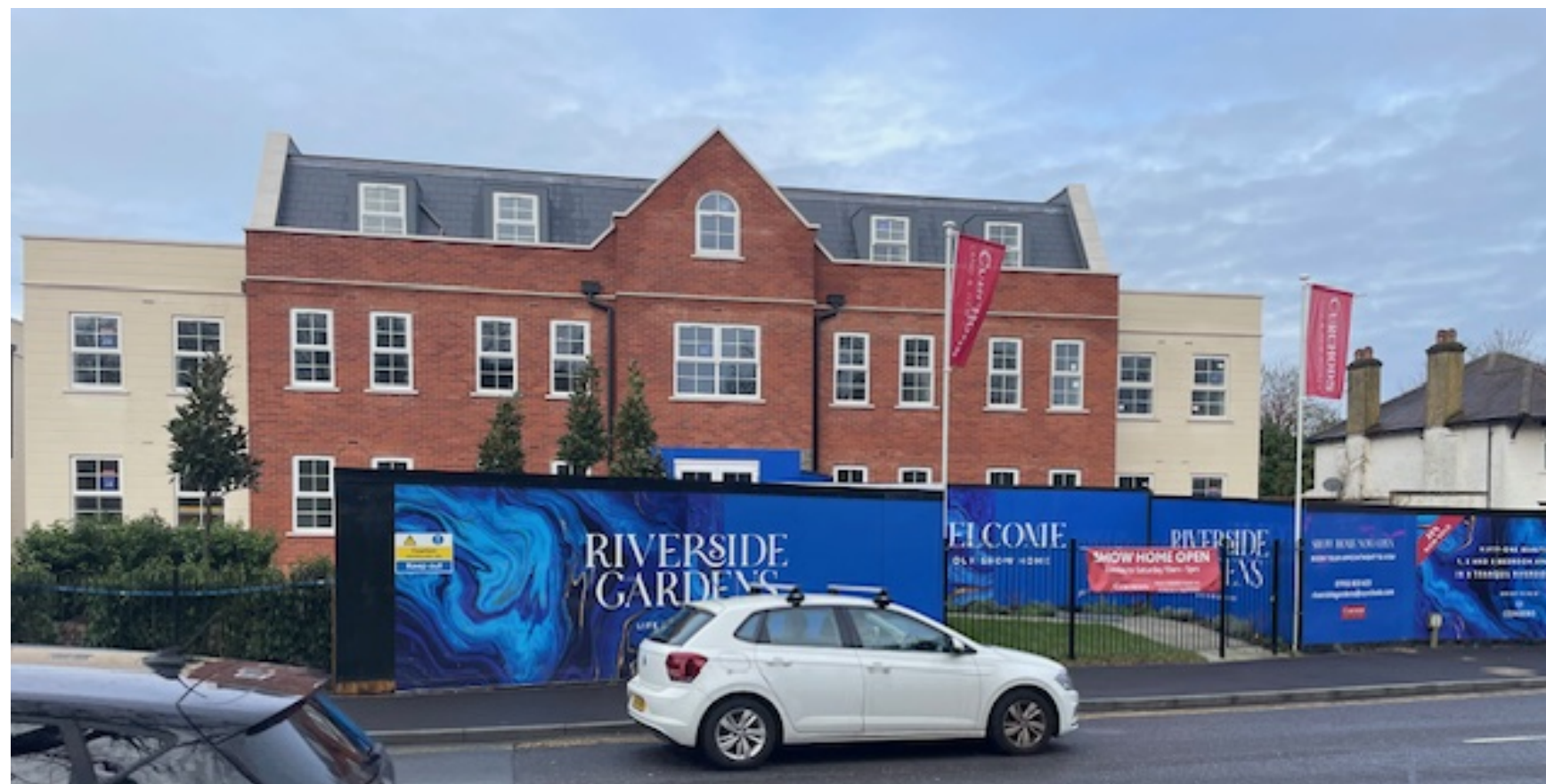
Riverside Gardens, 8-14 Oatlands Drive - Oatlands Drive elevation (under construction)
