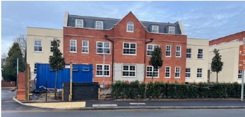
Riverside Gardens, 8-14 Oatlands Drive - Oatlands Drive elevation (under construction)
