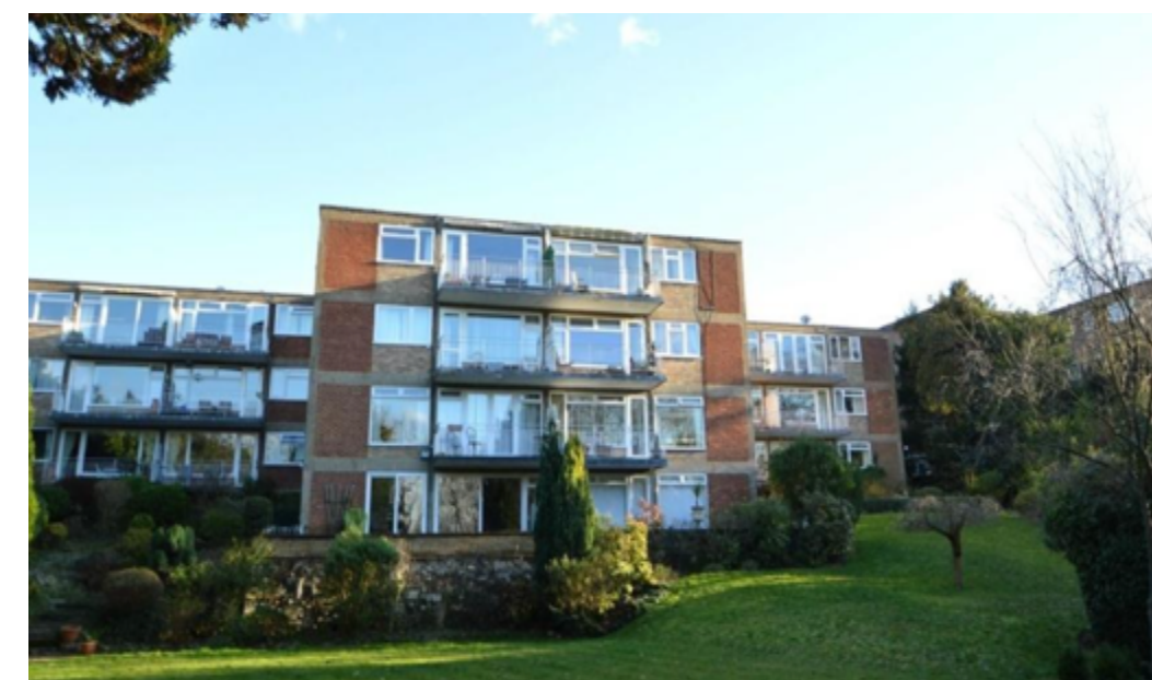
Chaseley Court, 42 Oatlands Drive - Rear elevation
