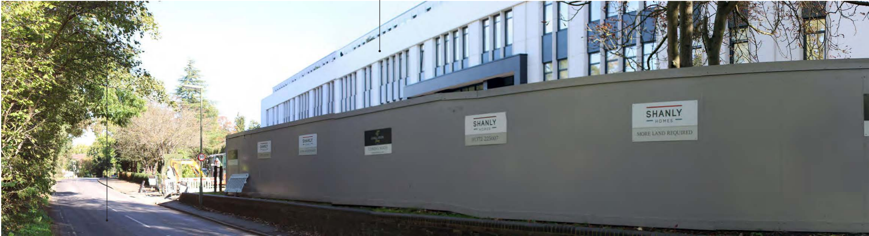
Photograph 18 View from Littleworth Road looking north east.
