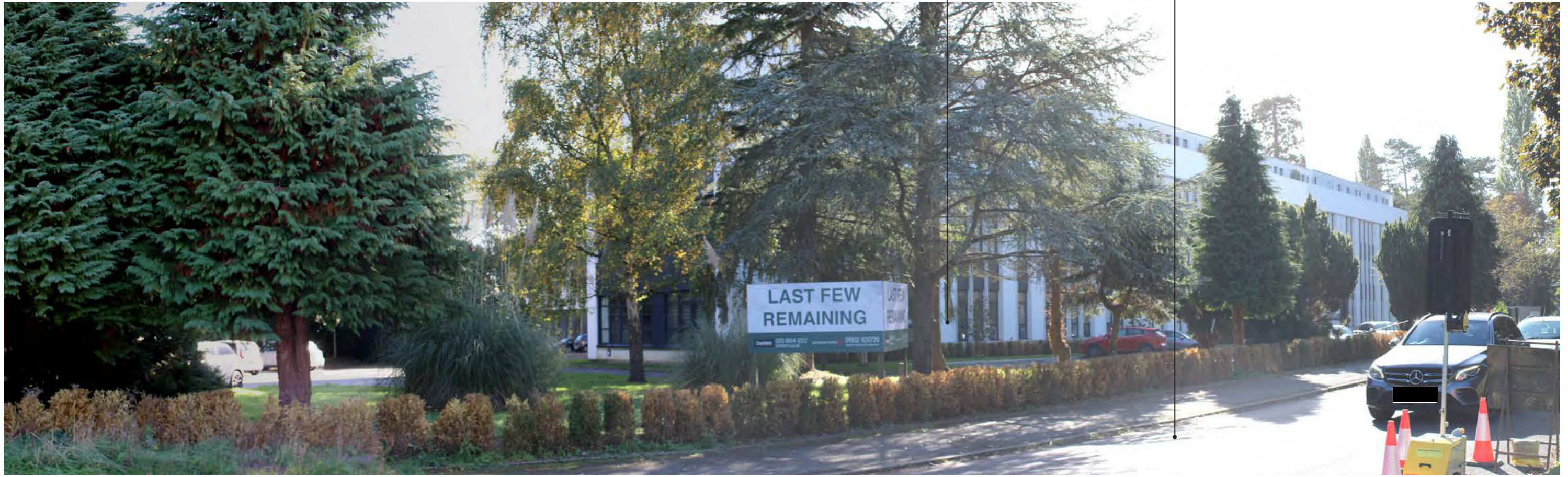
Photograph 19 View from Littleworth Road looking south east.
