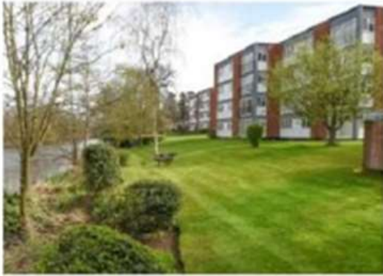
Berkeley Court - Rear elevation
