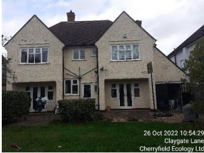
Figure 2: rear of B1
